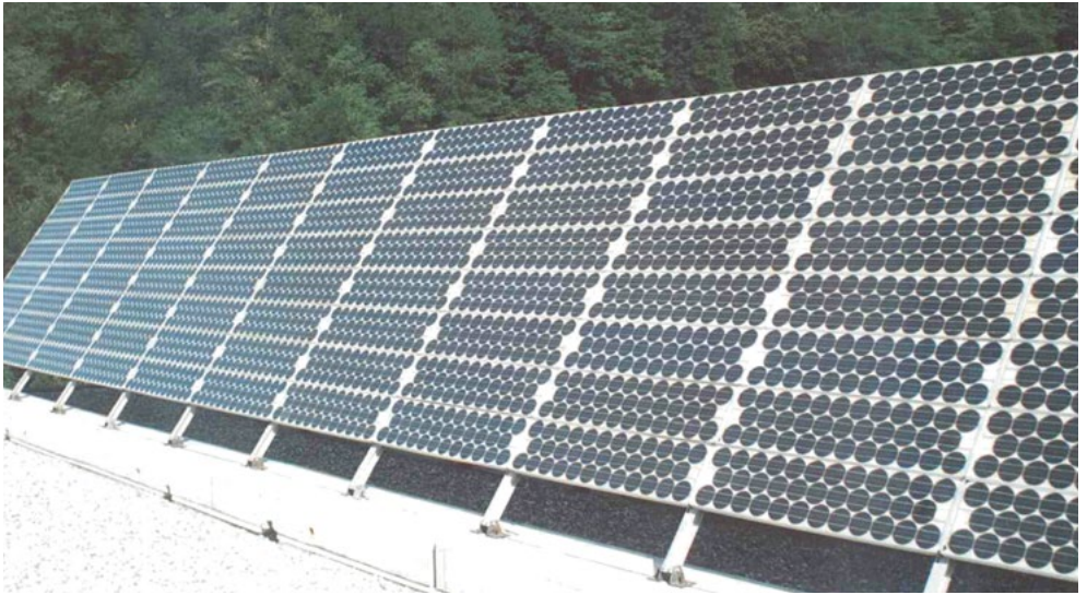
Fig. 05 LEFT. TISO - Inspection of the Ecopower inverter (1992) ©SUPSI Fig. 06 TISO - Configuration in 1995 ©SUPSI
