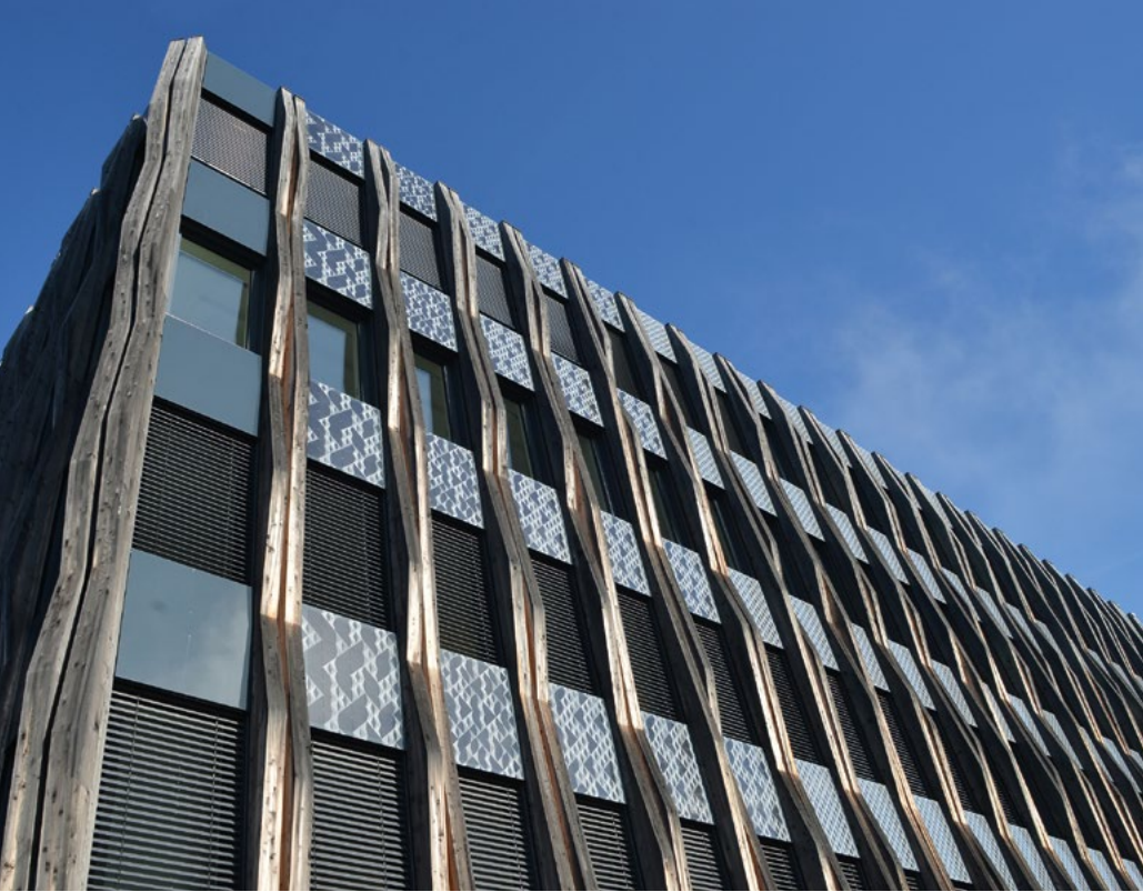
Fig. 42 ON THE PREVIOUS PAGE. Close up of the cSi and aSi photovoltaic façade of the Palazzo Positivo in Chiasso (Switzerland), by TUOR Baumanagement AG and Gasser Baumaterialien AG ©SUPSI Fig. 43/44 Z3 building of Ed. Züblin AG in Stuttgart, Germany. The design and the modules have been developed within the European project Construct PV ©SUPSI
