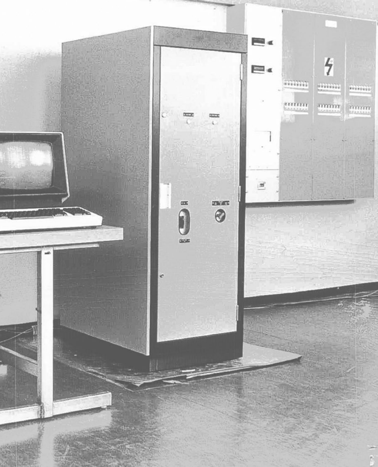
Fig. 01 ON THE PREVIOUS PAGE. TISO - Outdoor stand for the selection of modules (1981) ©SUPSI Fig. 02 TISO - First control room, with inverter and monitoring system ©SUPSI
