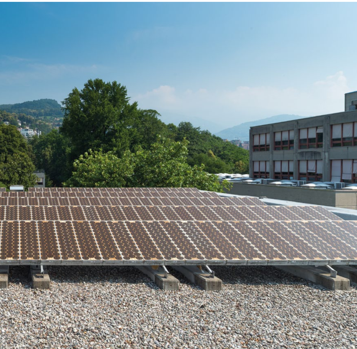
Fig. 13 TISO - panoramic picture of the 288 modules in the last configuration. The different classes of modules are well recognised from their colours ©SUPSI
