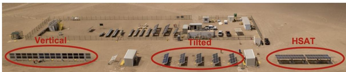
Figure 74: ATAMOSTEC Bifacial PV testing platform, Antofagasta, Chile
