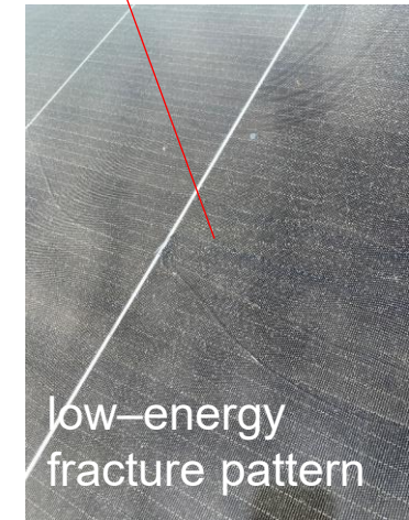
Repeated damage in same position: Shading induced?
